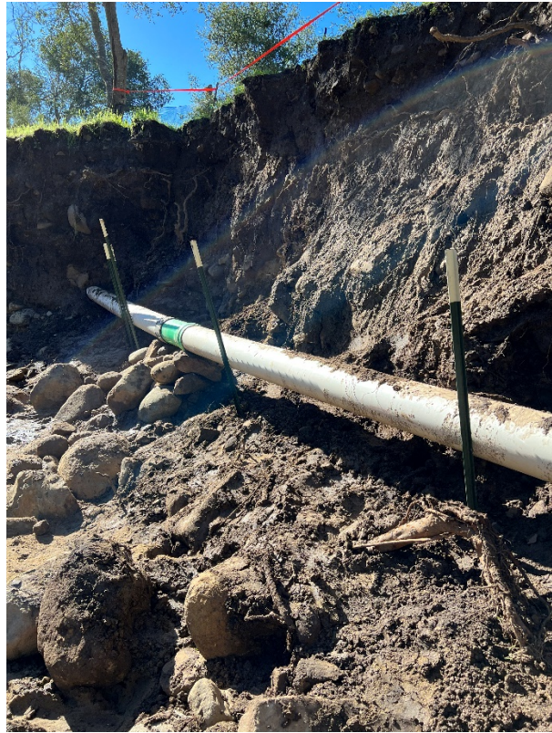
Photo 5: After Storm Pipe Repair
