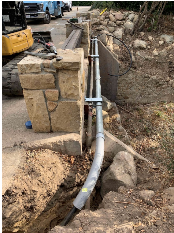
Photo 7: Before Storm (Prior to Backfill)
