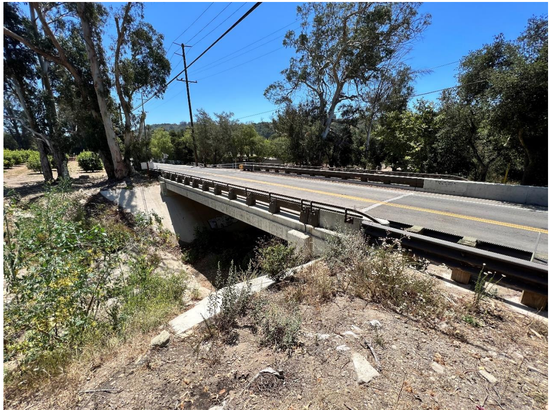
Figure 9.18 Romero Creek Crossing at East Valley Road/SR 192
