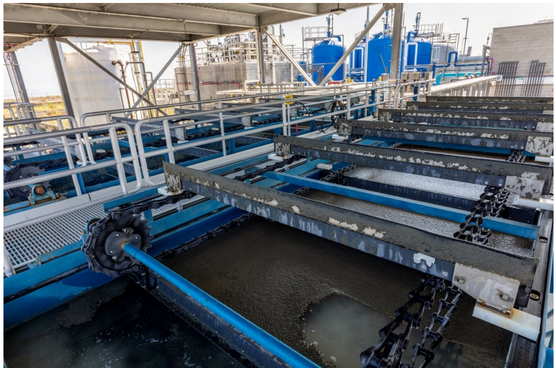
Figure 7.7 DAF Unit in Service
