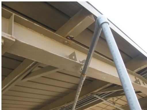
Photo 3.37 Chemical Storage Area Canopy
