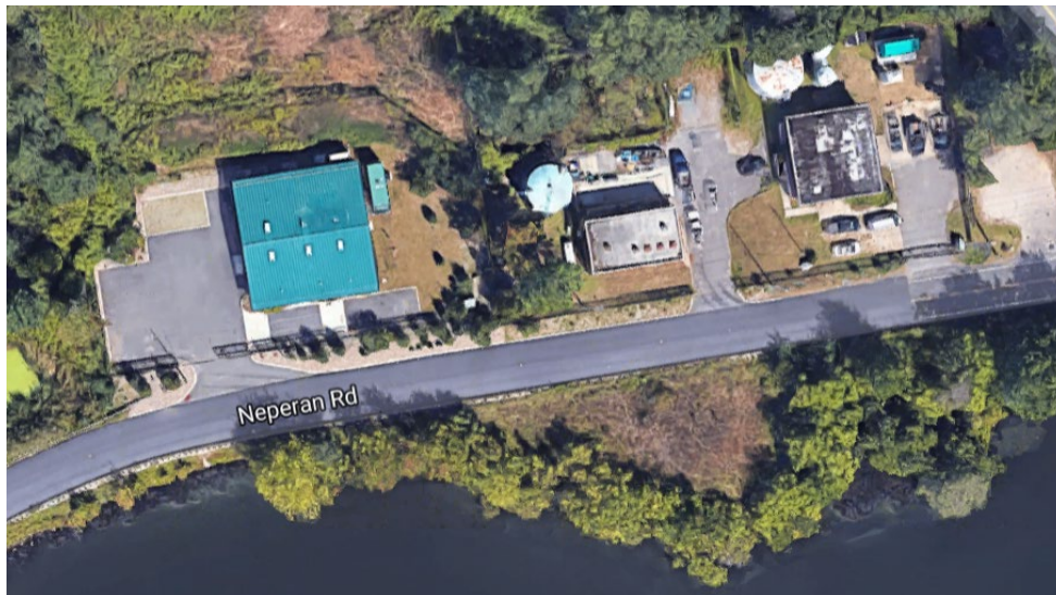
Picture: The three adjacent treatment and pumping stations of the Tri-Villages
