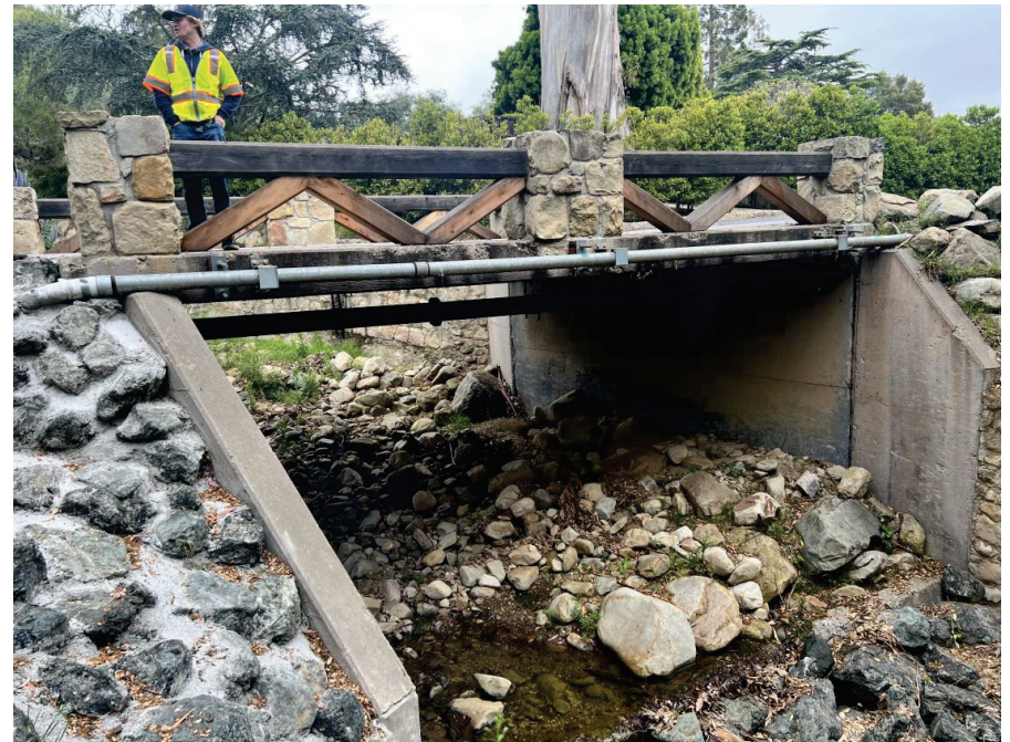
Existing Low Pressure Sewer System crossing Meadow Lane bridge (Riven Rock neighborhood)
