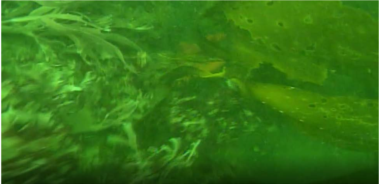
Photo of soft marine growth on outfall where riprap is not present
