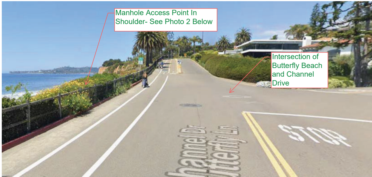
Photo 1: Area Surrounding Manhole Access Point
