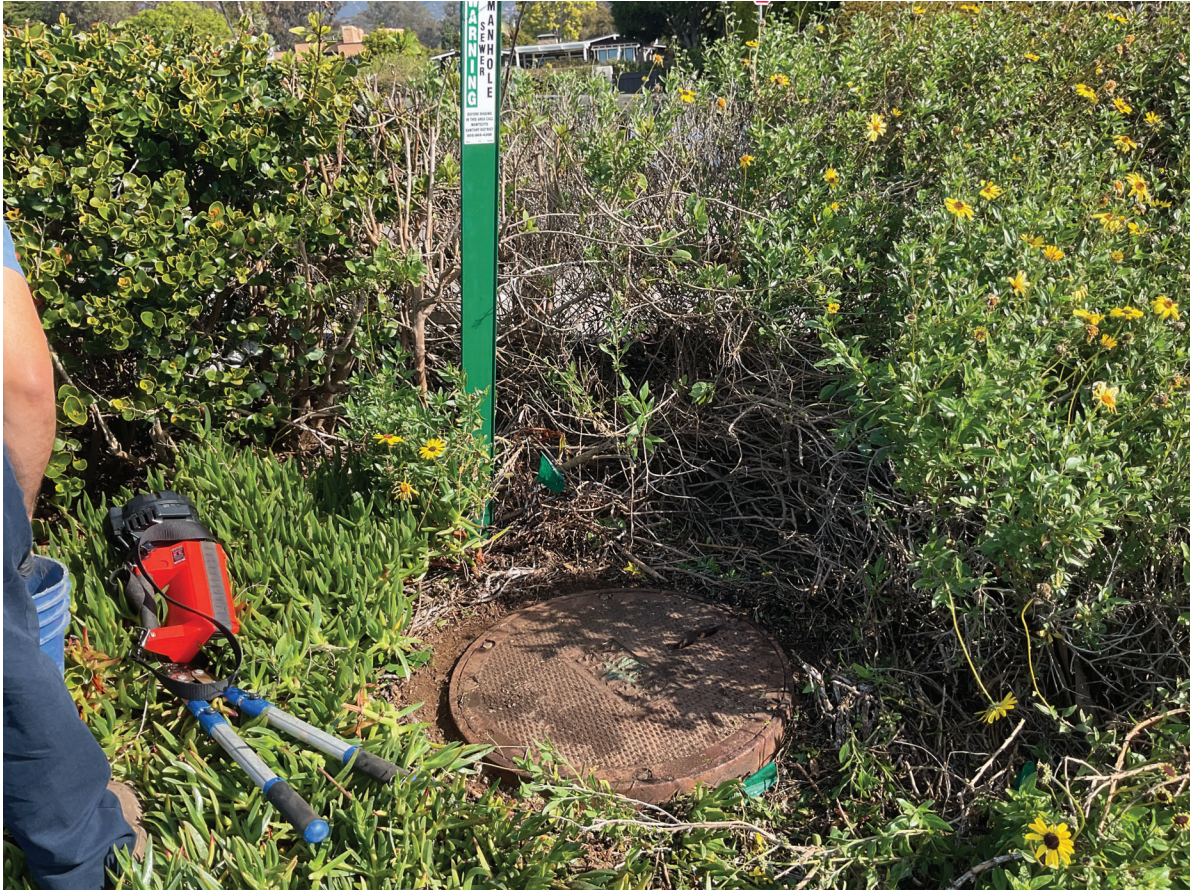
Photo 2: Manhole Access Point
