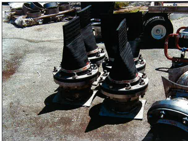
Photo 3 - Red valves bolted to saddles prior to installation.
