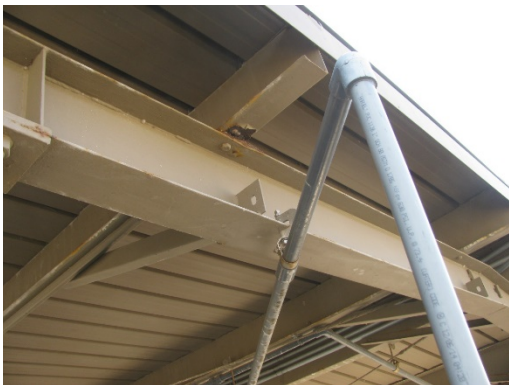
Photo 3.37 Chemical Storage Area Canopy
