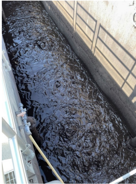
Photo 3.42 Aerobic Digester
