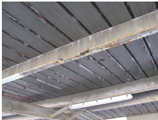
Photo 3.38 Sodium Hypochlorite Storage Facility Canopy
