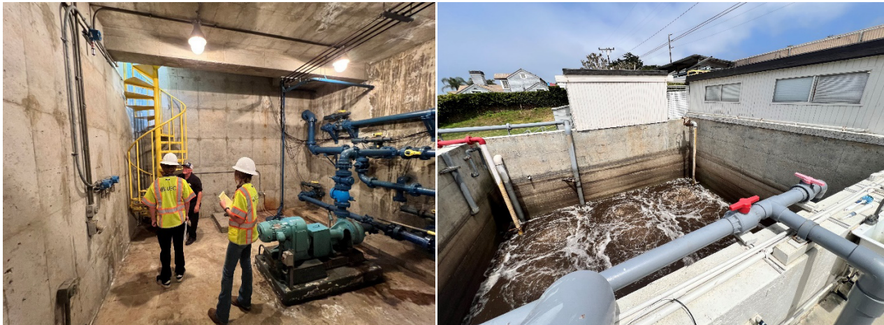
Figure 15 SSD WWTP Photos
