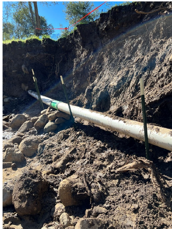
Photo 8: After Storm Pipe Repair
