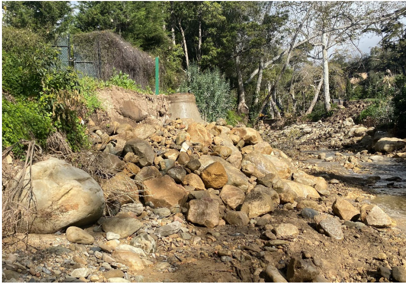
Photo 3: After Repair (Looking Upstream)
