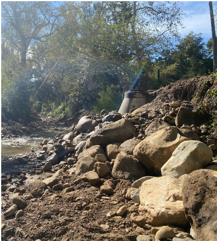
Photo 4: After Repair (Looking Downstream)
