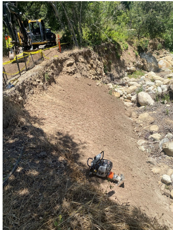
Photo 11: Final Cover (Looking Upstream)
