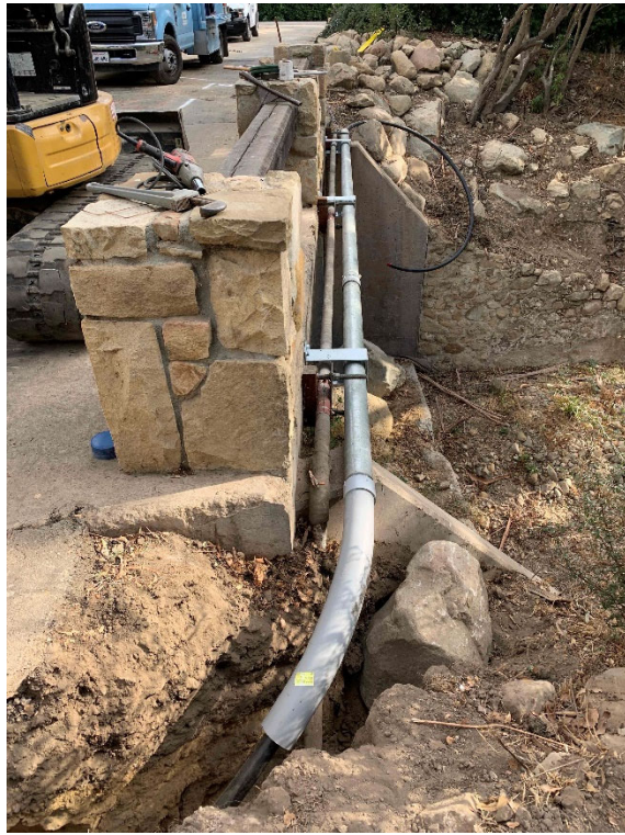
Photo 13: Before Storm (Prior to Backfill)
