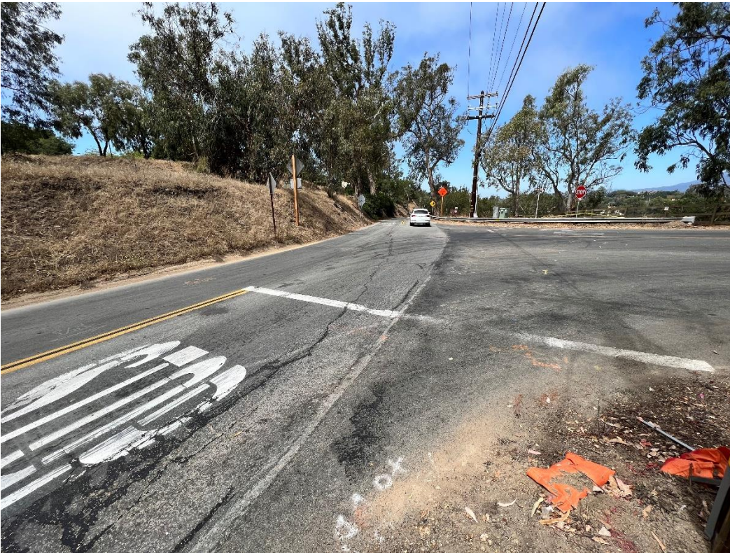
Figure 9.12 Ortega Hill Road Existing Utility Backdrop
