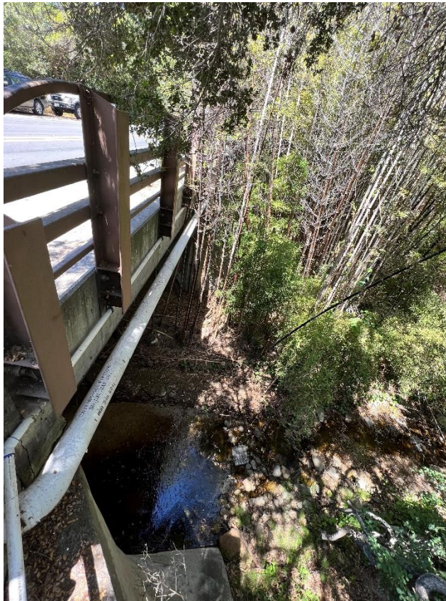
Figure 9.17 Romero Creek Crossing on Sheffield Drive
