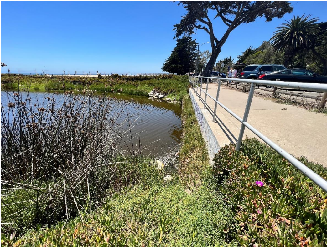
Figure 9.22 Culvert Crossing along Cabrillo Boulevard
