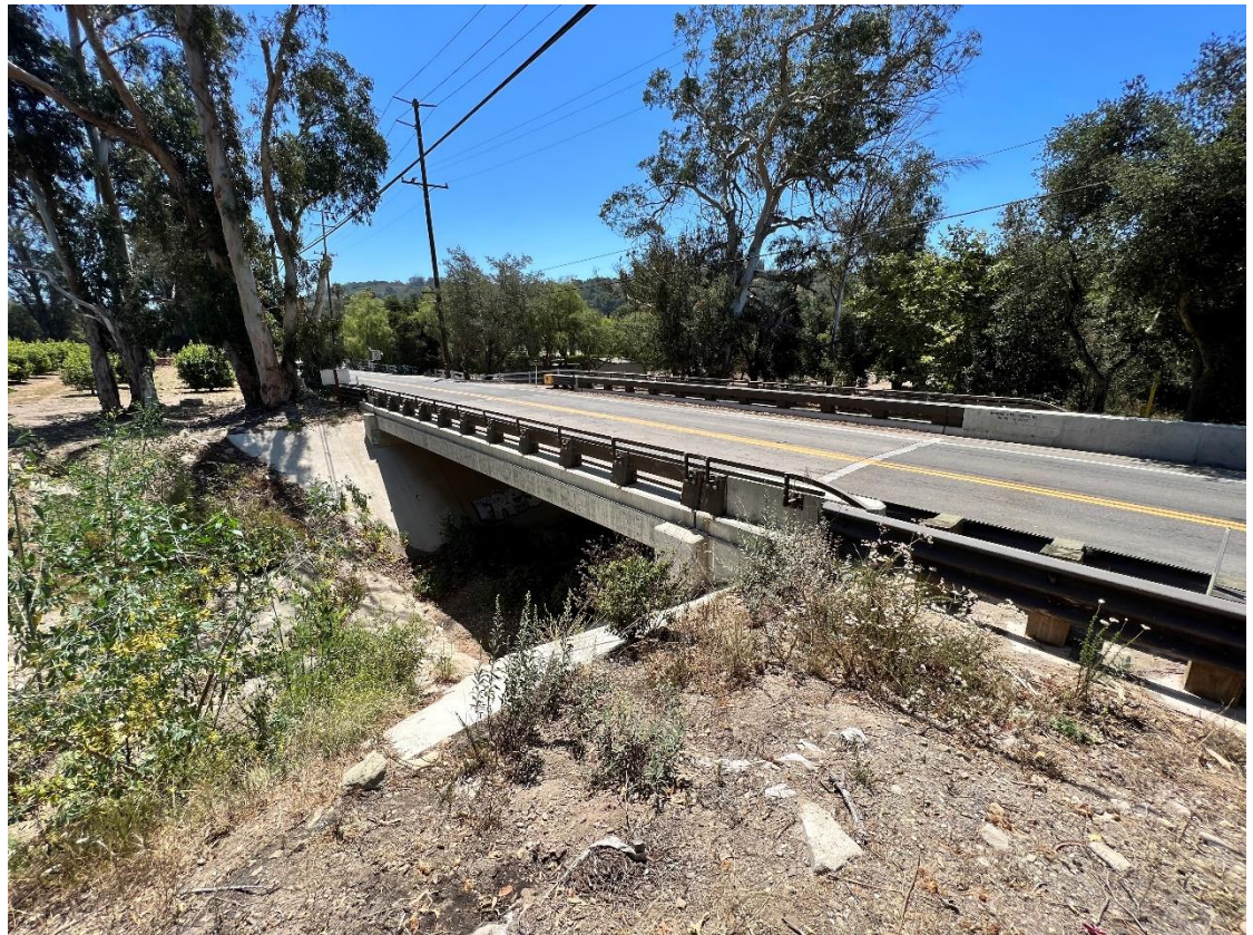
Figure 9.18 Romero Creek Crossing at East Valley Road/SR 192
